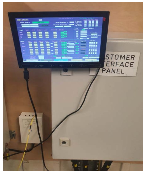
Figure 20: Power Potential achieves complex integration between DERMS, a DER and UK Power Networks' live network management system – verified during commissioning via displaying internal values on the Remote Terminal Unit's mimic.
