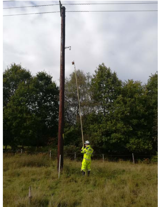
Figure 26: A Pathfinder being installed using magnetic mounts
