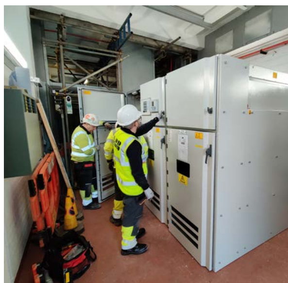
Figure 19: FLCB positioned into place and installation
