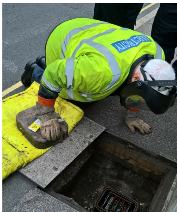
Figure 31: An old two-way link box
