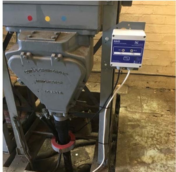
Figure 23: This Nortech NX45 fault passage indicator is battery operated and has a modem allowing remote communications to Network Control of other locations along an 11kV feeder, giving clarity of likely fault locations.
