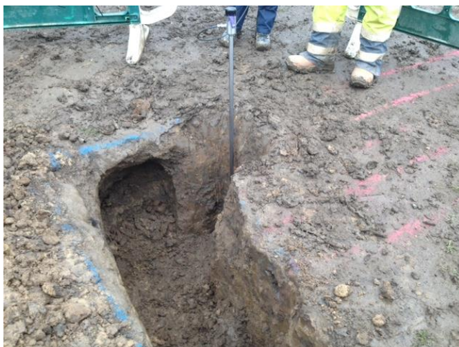
Figure 12: Thermal Resistivity measurements Source: J Murphy and Sons Ltd
