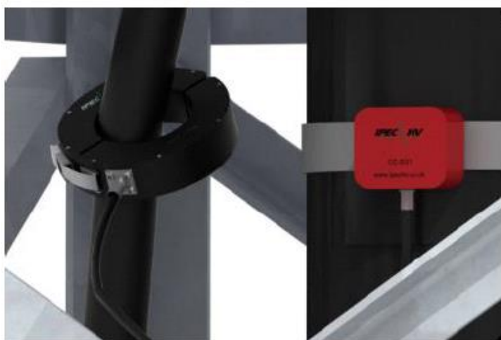
Figure 8: Partial Discharge sensors installed on a cable sealing end
