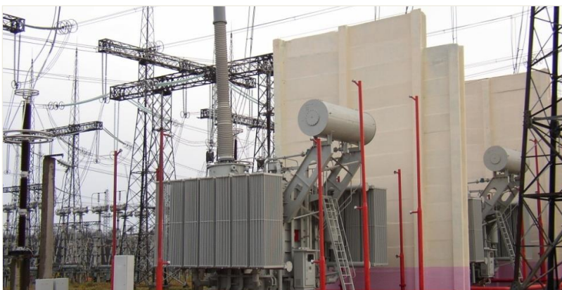
Figure 5: Magnetically Controlled Shunt Reactor (MCSR)
