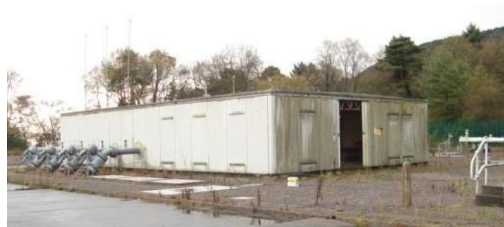
Regulator building at an Offtake
