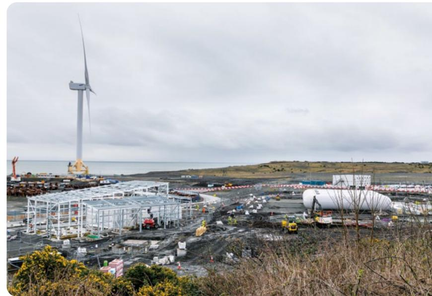
of six storage vessels were installed at the H100 Fife hydrogen production and storage site. The vessels will ensure the project can provide a constant source of hydrogen for even the harshest of winters.
