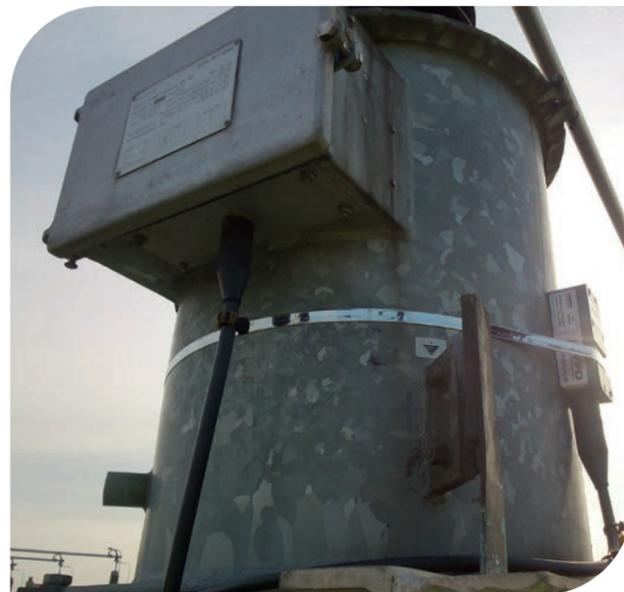
HVPD partial discharge monitoring sensor
