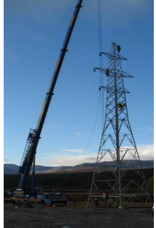
Figure 2 Conventional tower construction using crane
