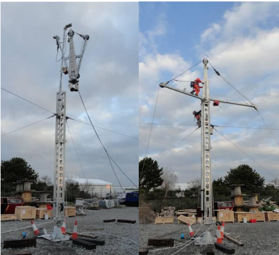
Figure 3 Alternative tower construction using emergency restoration system (ERS)
