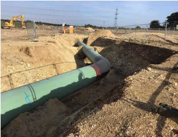
Example of pipeline considered for repurposing
