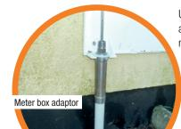
innovative push-fit adaptor has solved this issue, meaning the job can be done by one engineer. This reduces time on site and disruption to the customer and ensures we continue to deliver a reliable gas supply.
