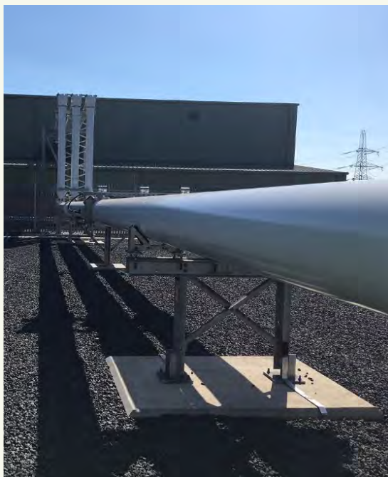
Outdoor section of 400 kV gas insulated busbar containing g3 gas.
