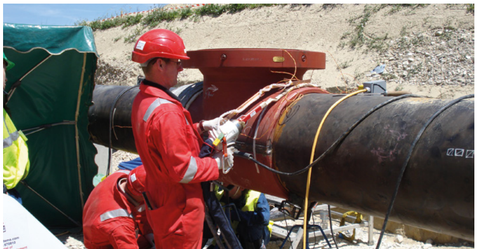
The wand will make the job of welding these fittings much safer.
