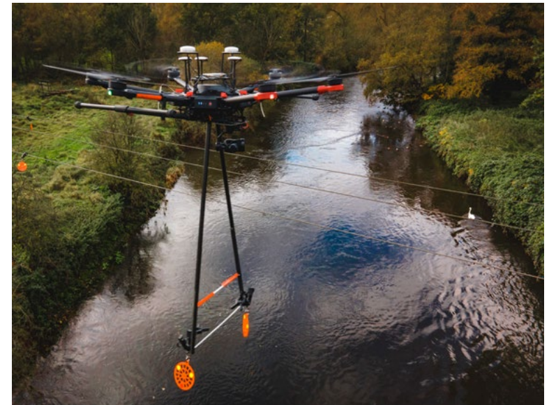
Figure 2: Drone installation of Bird Flight Diversers
