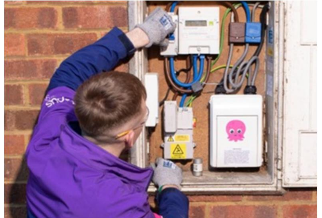
Octopus Engineer completing Emerge fuse upgrade
