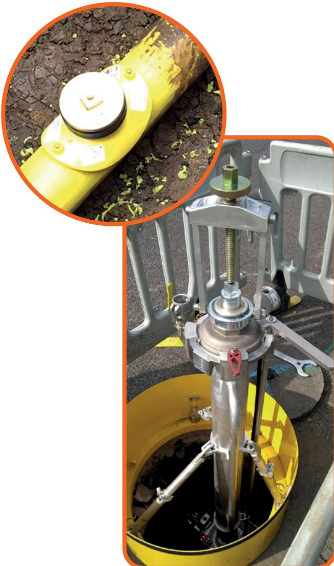
This NIA project (NIA\_SGN0093) allows use of an existing process and equipment by developing an appropriate electrofusion fitting to allow connection to the PE main and installation of the existing under pressure drilling machine and bag off equipment. The new fitting will be specifically designed to be compatible with not only the bag off equipment but will also allow use of the Synthocam 3 camera system and the I-branch water extraction tool.
