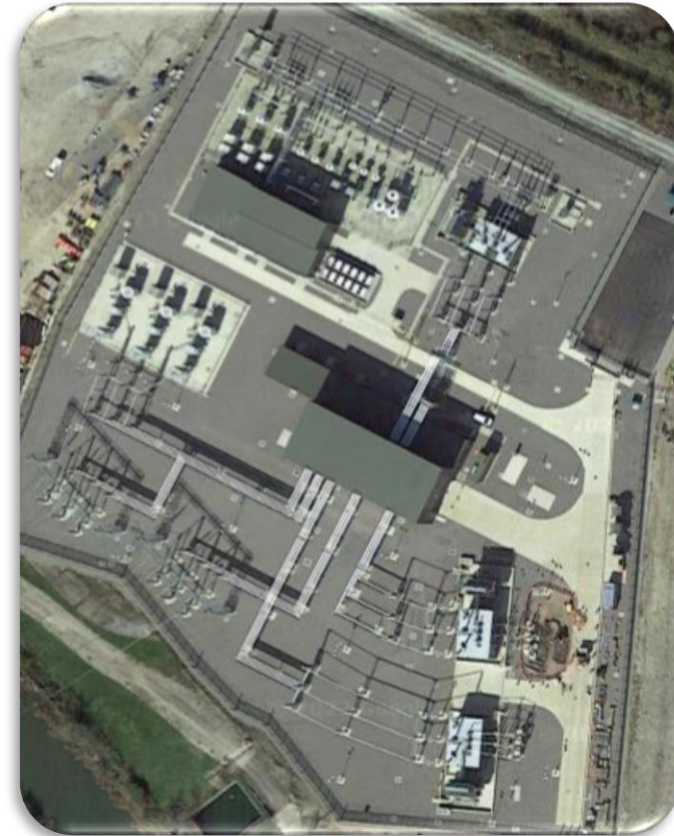
Substation B – relatively new
