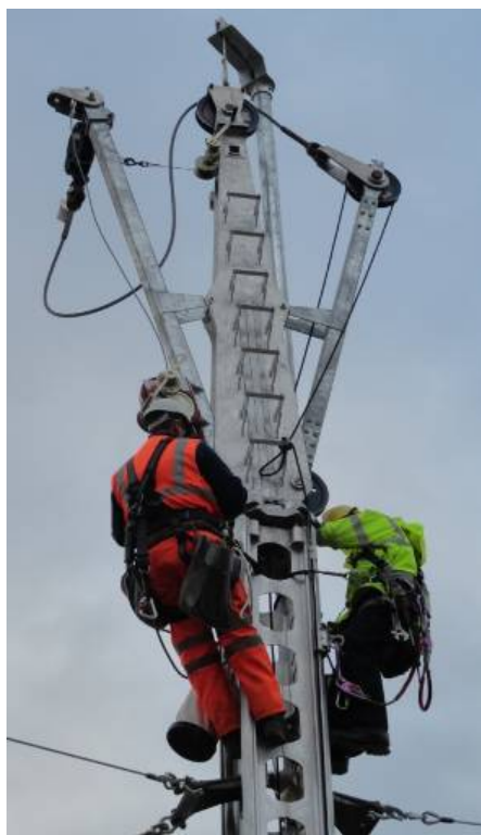
Figure 7. Training staff in the use of the modified Emergency Restoration System
