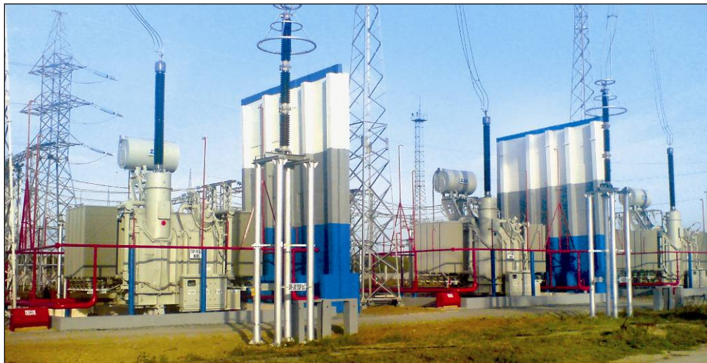
Figure 5. Magnetically Controlled Shunt Reactors (MCSR).
