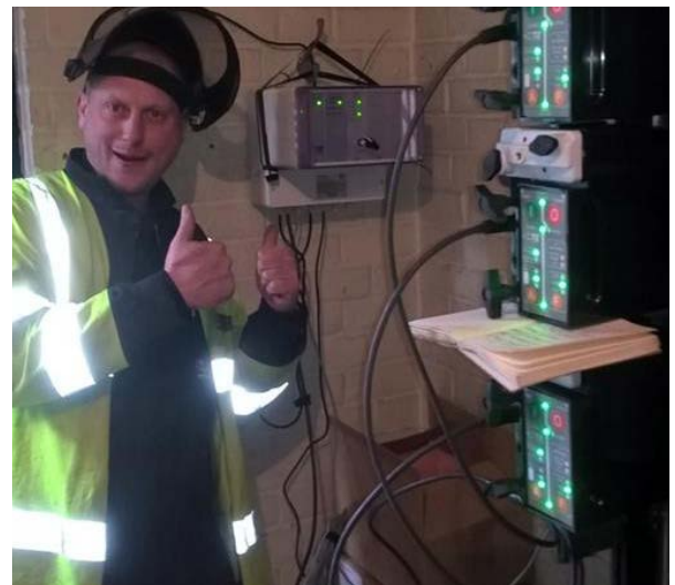
One of our London fault response team members checking out our new power electronics circuit breakers which will help us find faults faster and restore supply to customers quicker
