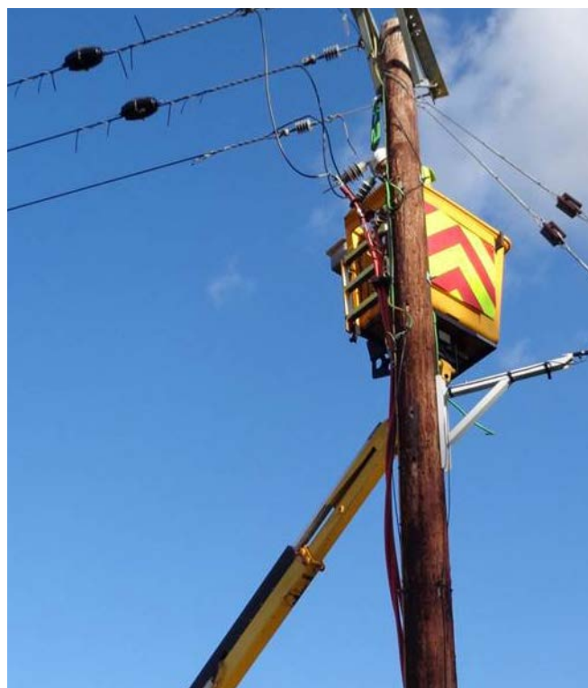
Early trial units for detecting broken or low hanging overhead line conductors being installed
