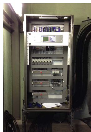
Dynamic Ratings E3 Transformer Management System (TMS), Weybridge Primary Substation
