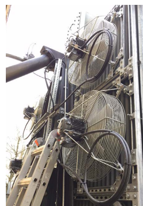
Additional Transformer Cooling Fans, Weybridge Primary Substation
