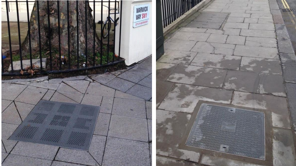
Figure 8: Composite vented Cover (Left) and non-vented cover (Right)
