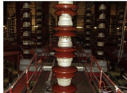
It is proposed to extend the safe working area to encompass all 9 stacks which make up the isolator. This will however necessitate the need to develop a bespoke hand rail mechanism. In Photo 1 there is a need to maintain the physical separation between the MBB Isolator on the right and the RBB isolator on the left. At this point the hand rail will be required to be a bespoke engineered solution for the following reasons.
