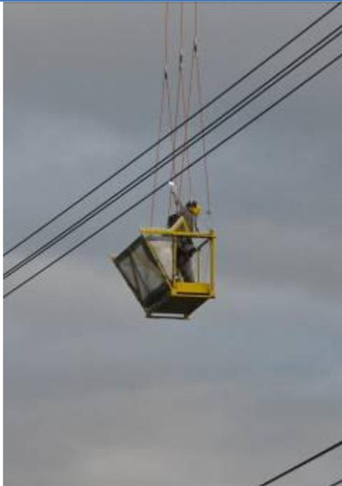
**Figure 8 – Linesman Bonding onto Live Conductor**
