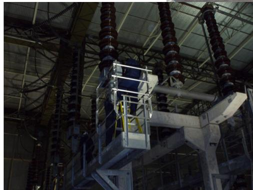
Another major issue is the maintenance of FMEs at height. This has previously involved utilizing a step ladder while already at height. The development and trialling of an access platform and extended handrail system as pictured above should reduce the inherent risk of these maintenance activities.
