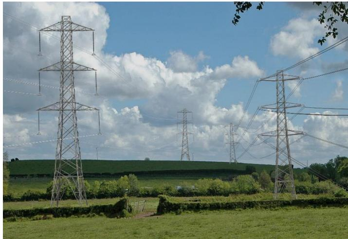
Photo-montage of 275kV standard tower and a reduced height tower fitted with insulating cross-arms
