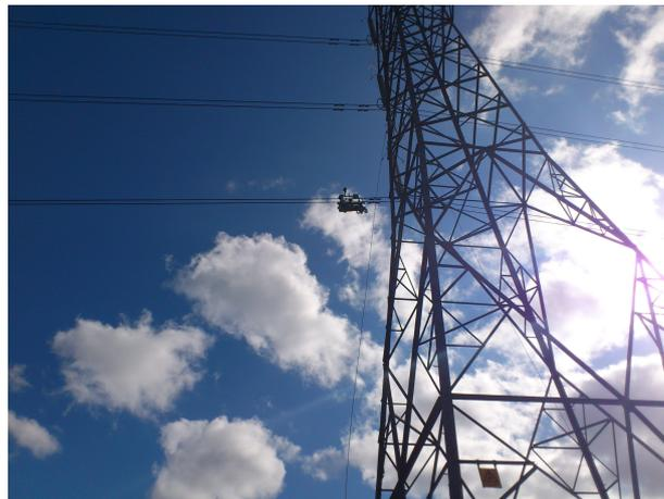
During 2012, as part of National Grid's preparations for the London Olympics, Hydro Quebec was asked if they could demonstrate the capability of the robot in repairing a number of defects on an inaccessible Earthwire associated with a circuit feeding into an Olympic venue. This type of repair had not previously been undertaken and National Grid worked in collaboration with Hydro Quebec on a solution.
