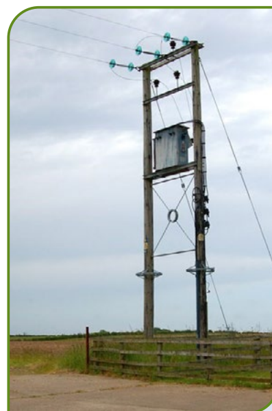
Pole Mounted Transformer
