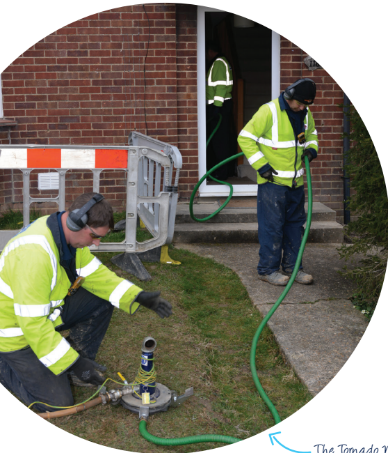
The Tornado Max adaptor being used to remove trapped gas safely
