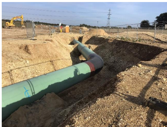
Example of pipeline considered for repurposing
