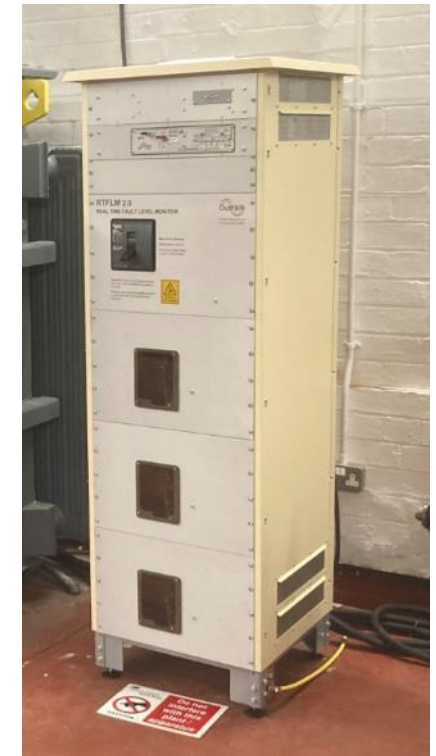
Real Time Fault Level Monitor at Sheil Park Primary, Liverpool, 2023
