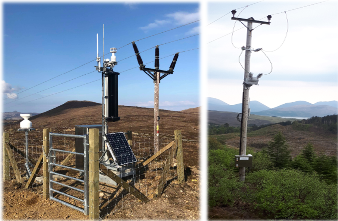
Figure 20. Left-hand picture is the stand-alone gateway powered by a solar panel, a vertical wind turbine and a car battery and the right-hand picture shows power tapped using a voltage transformer to feed a pole mounted gateway.
