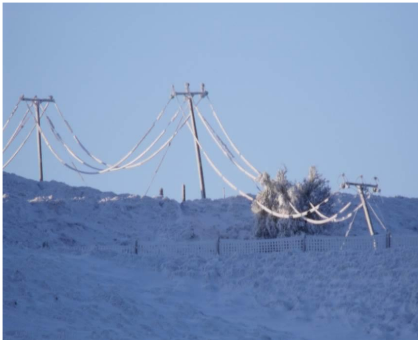
The effect of severe ice loads on an 11KV overhead line in winter 2010. STP Module 2 Project S2164_1 is looking at designs for future ice accretion and wind loads.
