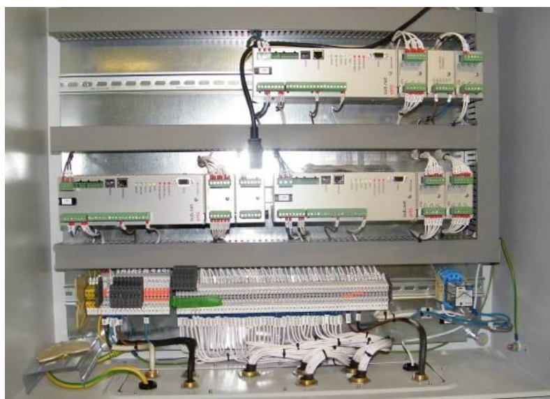
Disturbance recorders installed at the 132/33kV source substation to act as remote current monitors on the three 33kV feeders, which supply the unbalanced meshed network
