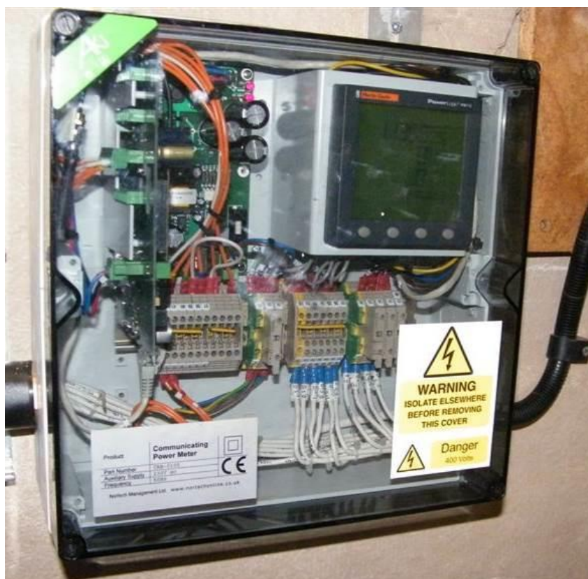
One of the remote Communication Power Units monitoring an 11kV site with embedded generation.
