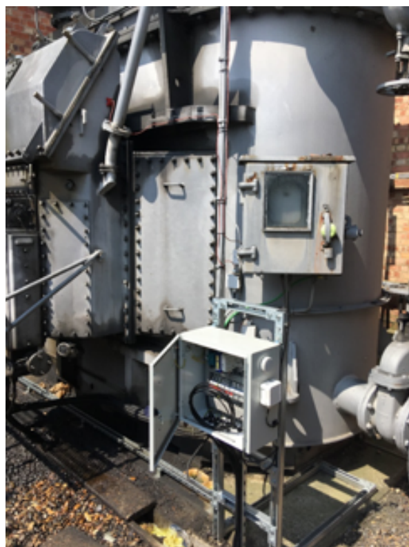
Figure 8 – Dissolved Gas Analyser Installation in Wickford Primary Substation
