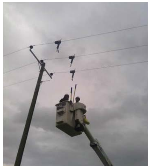
Insulation of an Aclara power sensor
