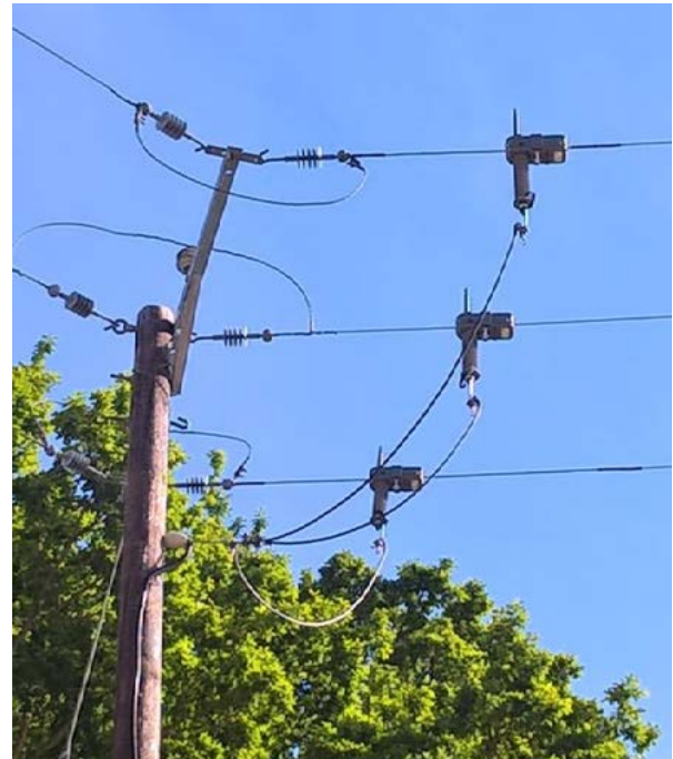
Aclara power sensors connected to 11kV overhead conductors
