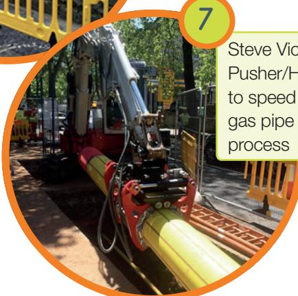
7 Steve Vick's Pipe Pusher/Handler to speed up our gas pipe insertion process
