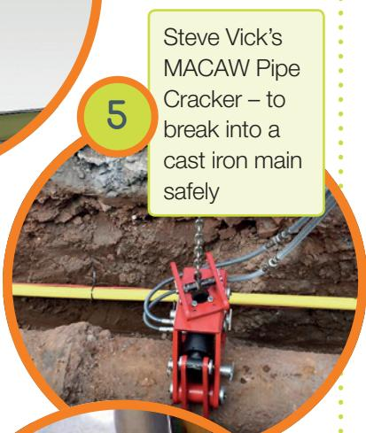
5 Steve Vick's MACAW Pipe Cracker – to break into a cast iron main safely
