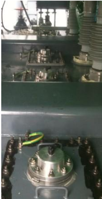
View along the line of four UHF window sensors on top of the tank.
