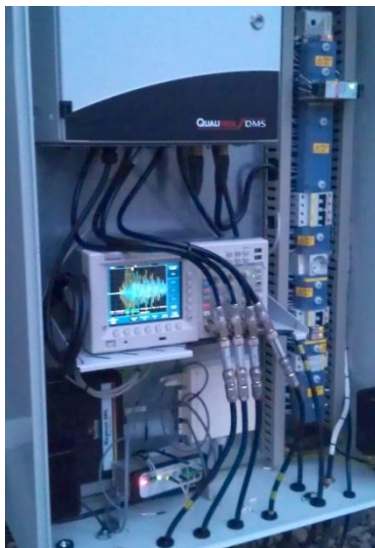
Equipment cubicle adjacent to the transformer. UHF cables enter at the bottom. Four of them feed into the oscilloscope before connection to the Qualitrol PD monitor.
