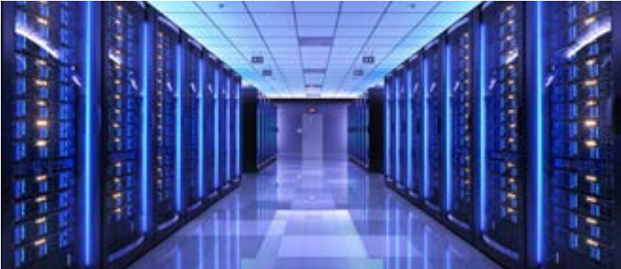
Figure 21: Infrastructure has been deployed across all three of UK Power Networks’ licence areas
