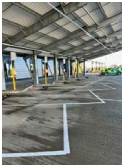
Figure 8: Electric charging bays for East of England Ambulance Service
